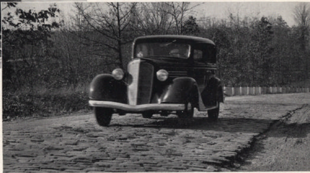
THIS IS THE FAMOUS Belgian Block Road at the General Motors Proving Ground. It is constructed of granite blocks laid irregularly on a 6-inch concrete base. On this unusually rough stretch Buick's smooth, gliding ride was put to one of its severest tests . . . and came through with colors flying!
